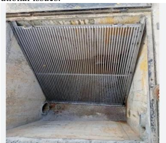
Figure 4.1 Coarse Bar Screen Chamber
