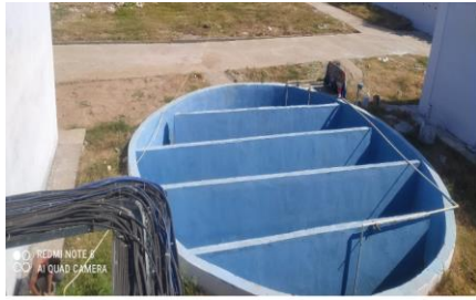
Figure 4.8 Chlorine Contact Tank
