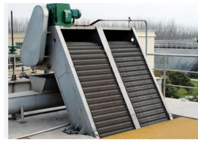
Figure 4.3 Fine Bar Screen (mechanical)
