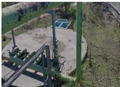
Figure 4.2 Collection Sump Tank
