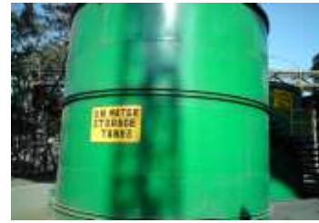
Figure 3.11 DM Water Storage tank-3 of capacity 100KL
