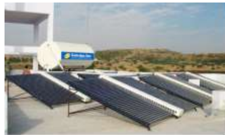
Figure 3.4 Solar Arrays of capacity 500 Liters each
