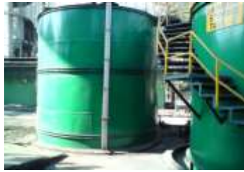
Figure 3.10 DM Water Storage tank-2 of capacity 100KL
