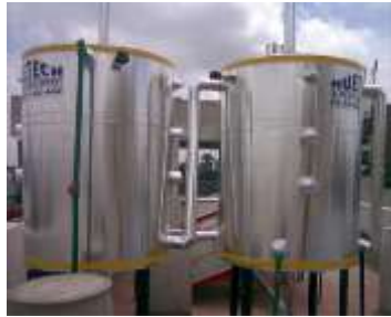
Figure 3.5 Solar Water Storage Tank
