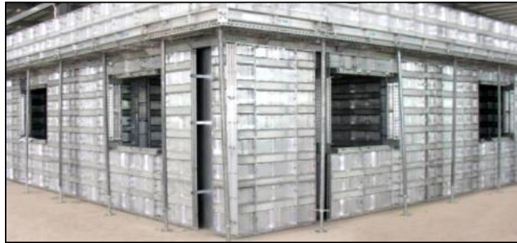
Fig no. 1 – Aluminium formwork system
