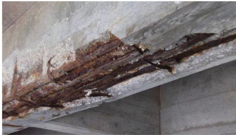
Figure 1.1: Deteriorated RC Beam in Practice
