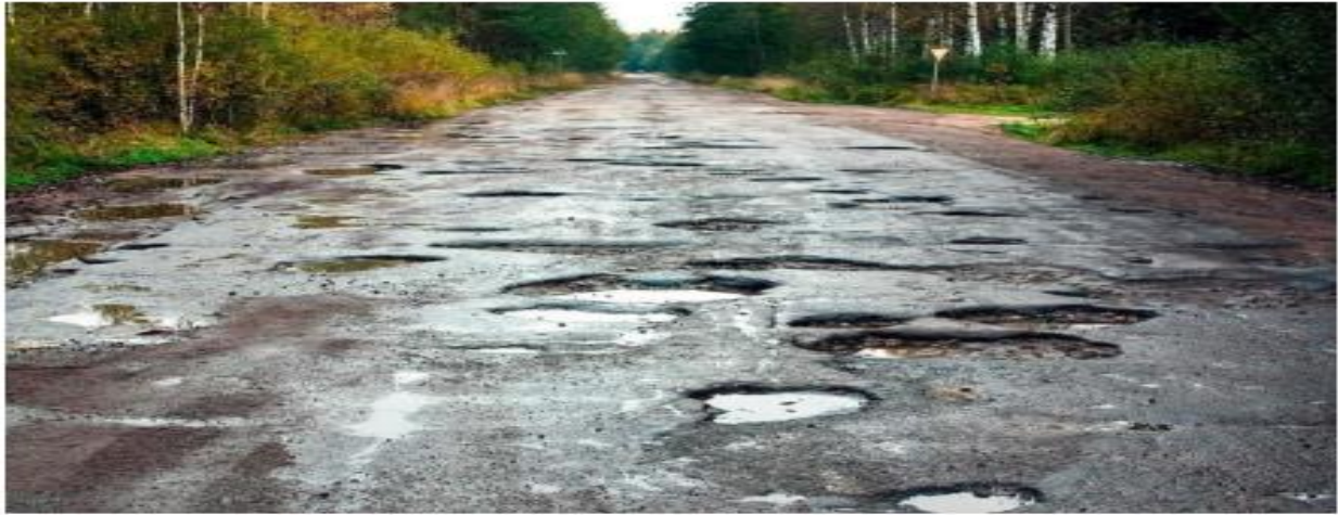
Figure 1 : Potholes on the Road
