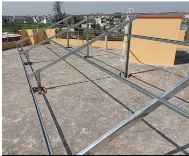
Figure4 GI roof top structure
