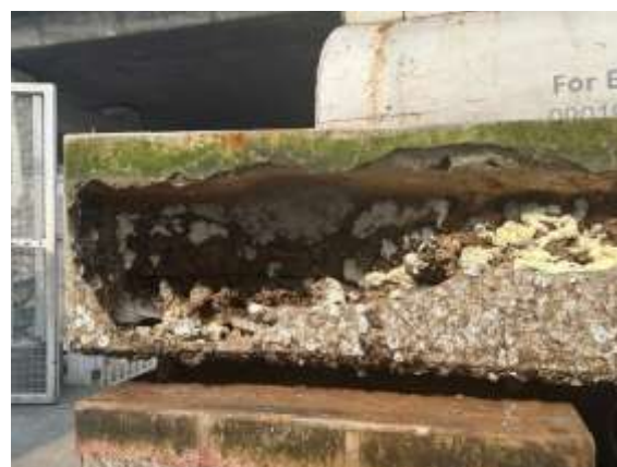
Figure 20: Damaged concrete pontoons due to prolonged water exposure
