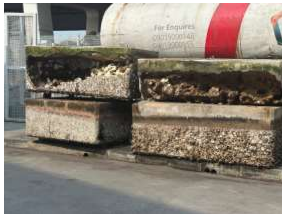
Figure 19: Stacked disused pontoons due to prolonged water exposure at Five Cowrie terminal
