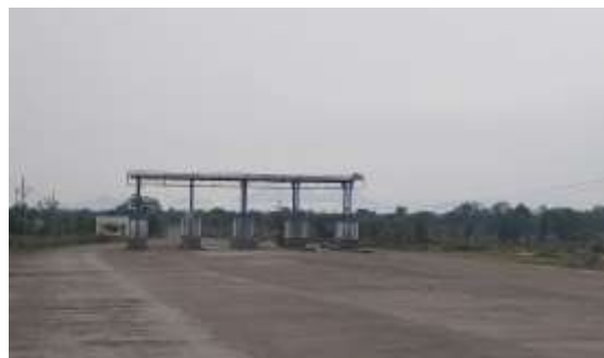
Fig-IV Lack of signboards and marking in approach of Toll Gate
