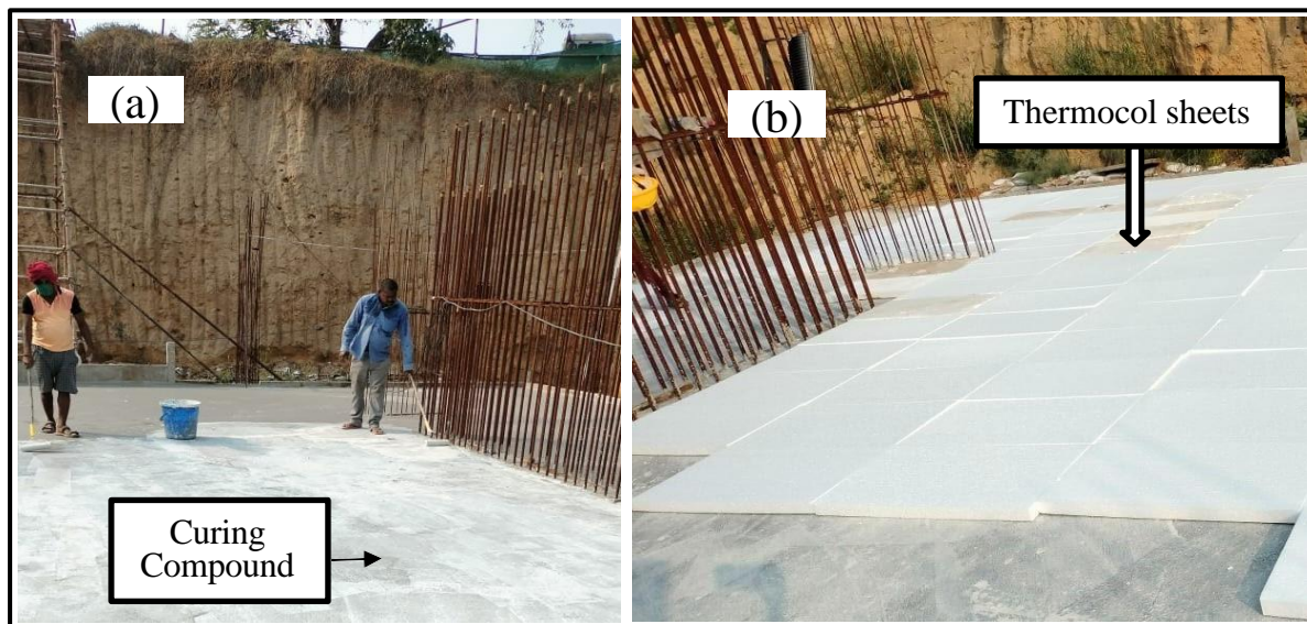
Fig - 2: (a.) Application of curing compound in progress at the site (b.) Laying of thermocol sheets over the curing compound at the site
