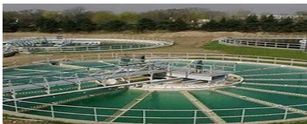
Fig-01 – Circular Sedimentation Tank
