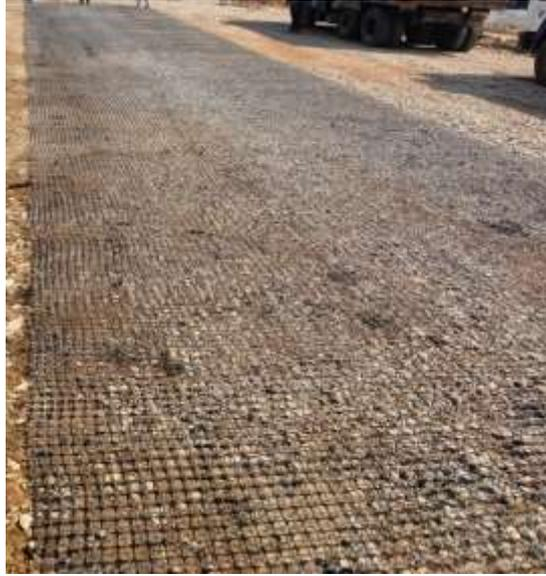
Figure 6: Fixing of Bi-axial Geogrid Over GSB Top Layer
