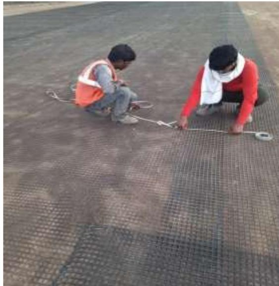
Figure 5: Fixing of Bi-axial Geogrid Over Subgrade Top Layer
