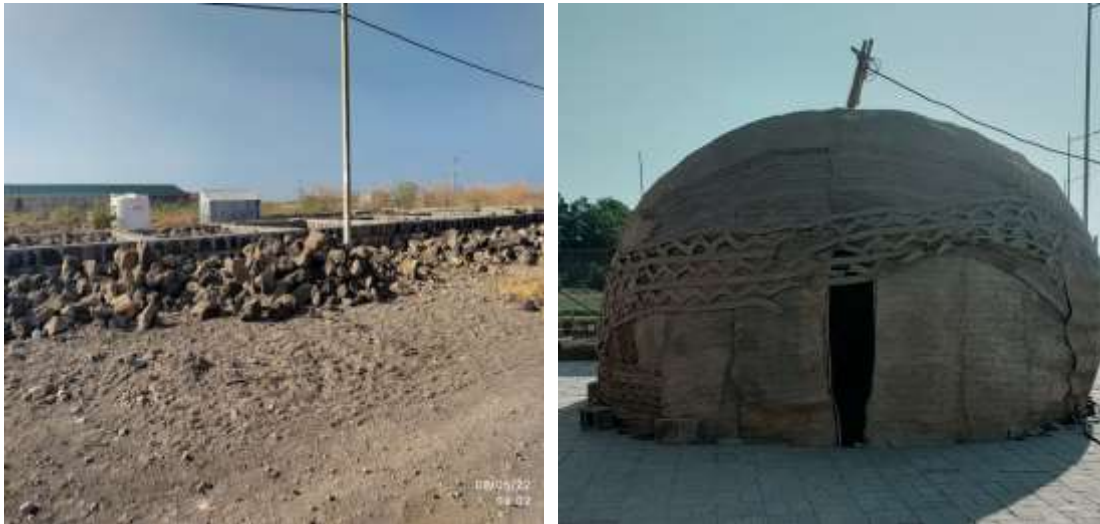
Figure 1. Construction of structure using locally available stones, mud and bamboo (Source: Author)
