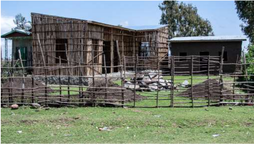
Figure 2. Construction of houses using bamboo. (Source: Google)
