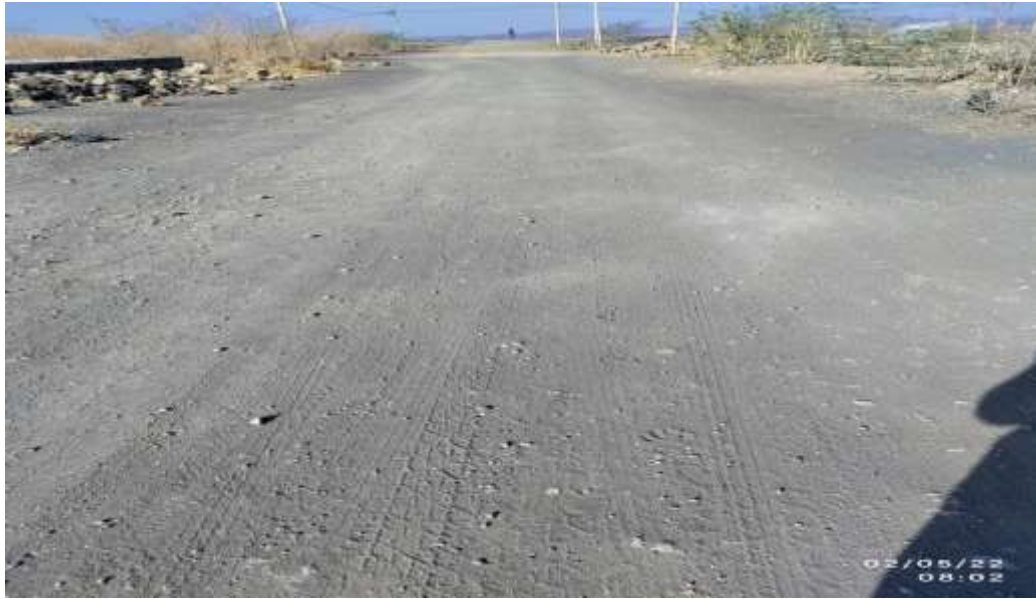
Figure 4. Collector road made from compaction of locally available materials. (Source: Author)
