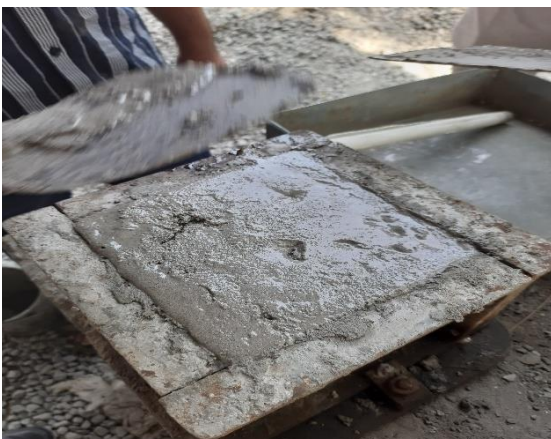
Fig -1: Concrete Cubes casting
