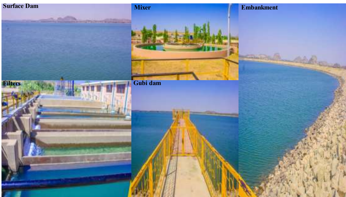
Figure-1 In this figure includes the components like a Surface Dam, Mixer, Filters, Gubi Dam and Embankment within a water treatment system context flow and treatment process of water from the Gubi Dam reservoir to the distribution network.
