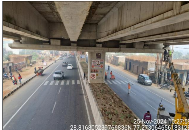
Figure 1 General view of bridge
