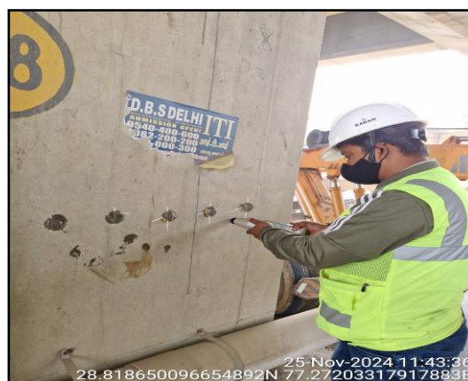
Figure 4 Rebound Hammer Test
