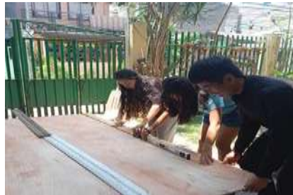
Figure 2: Construction of a foundational structure
