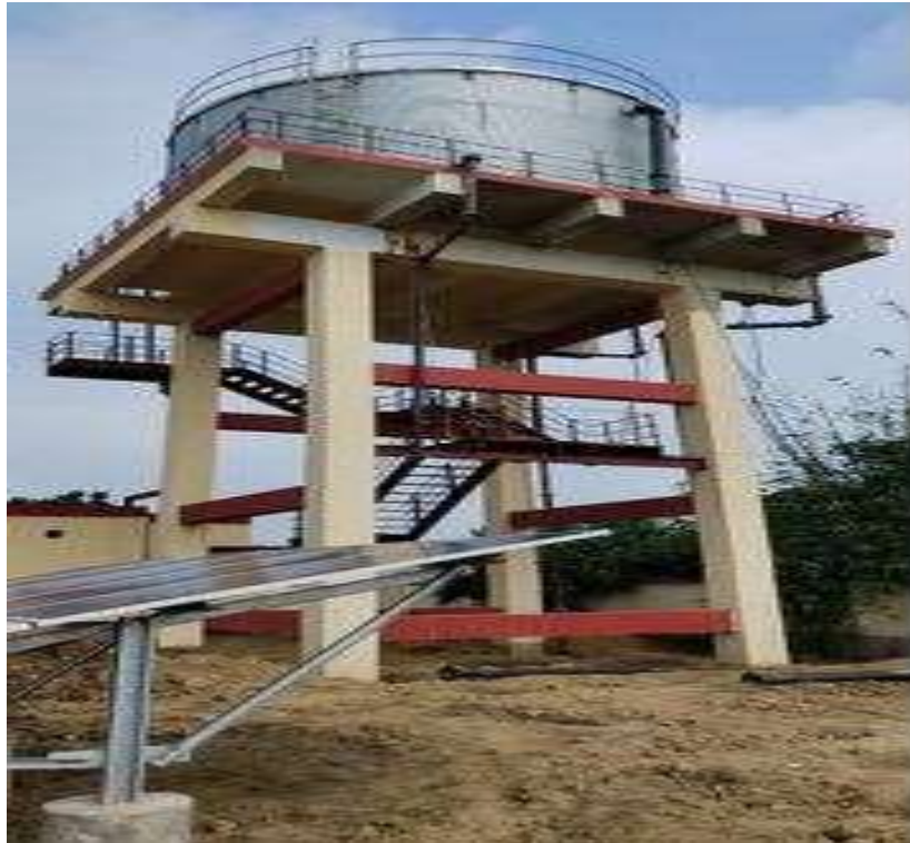
Figure 1 Water tank resting on sloping ground
