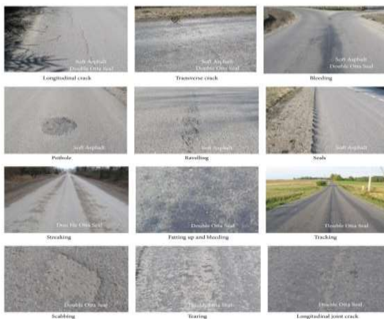
Fig.2:Different defects in asphalt pavement
