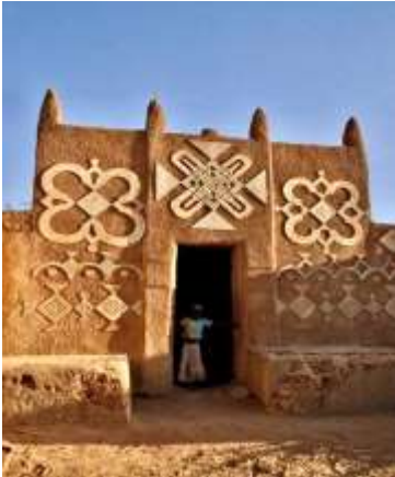
Figure 4: Traditional Hausa Facade Decoration showing Pinnacles (Zankwaye).
