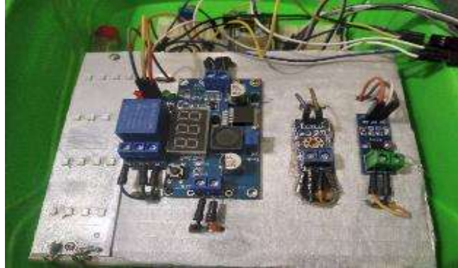
Fig. 17 Power Monitoring Circuit view
