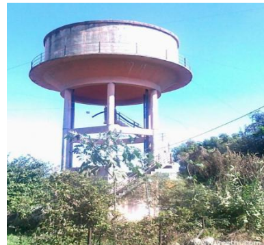
Figure 1.6 Overhead water tank floor
