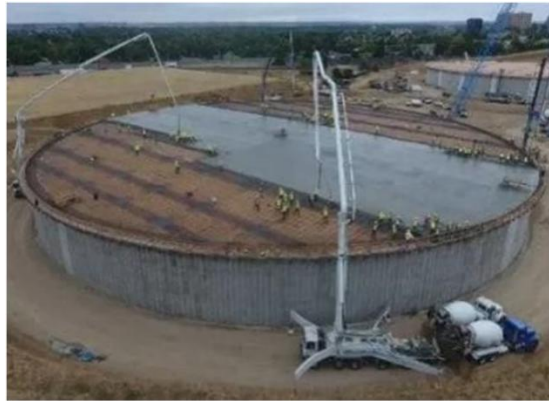
Figure 1.9 RCC water tank roof
