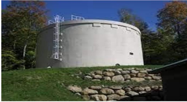
Figure 1.1 RCC water tank on earth surface
