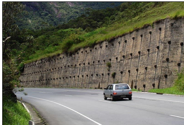
Fig 1 Roadside Retaining Wall
