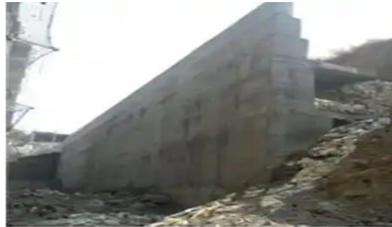
Wall at Location : Dhayari Pune
