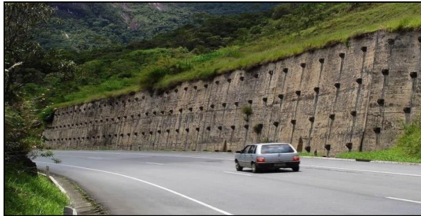
Fig 1 Roadside Retaining Wall
