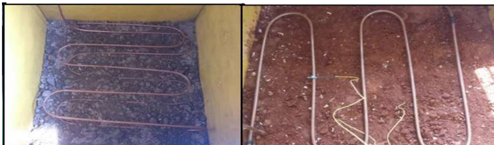
Fig 1.2: Placement of Earth Tubes
