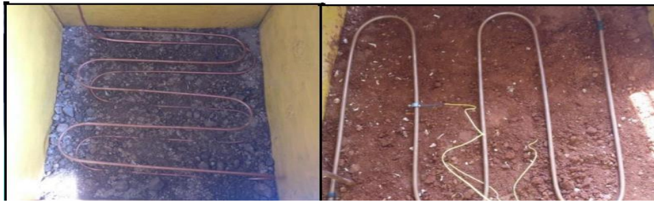
Fig 1.2: Placement of Earth Tubes
