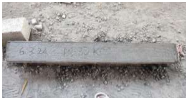
Fig. 9 – Casting of beam
