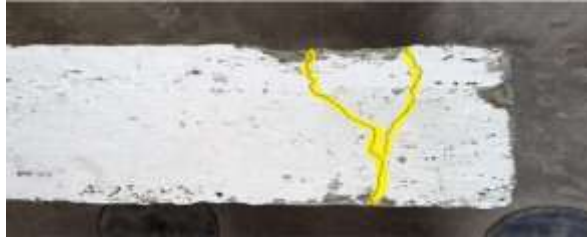
Fig 15: Crack on conventional column specime
