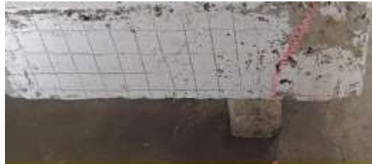
Fig 13: Crack on conventional column specimen
