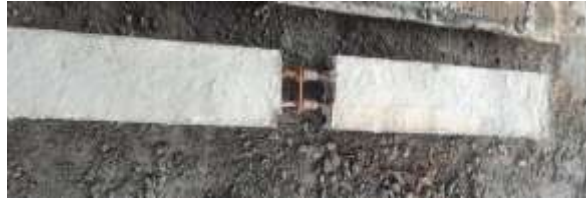
Fig 2: Casting of coupler in column-to-column connection
