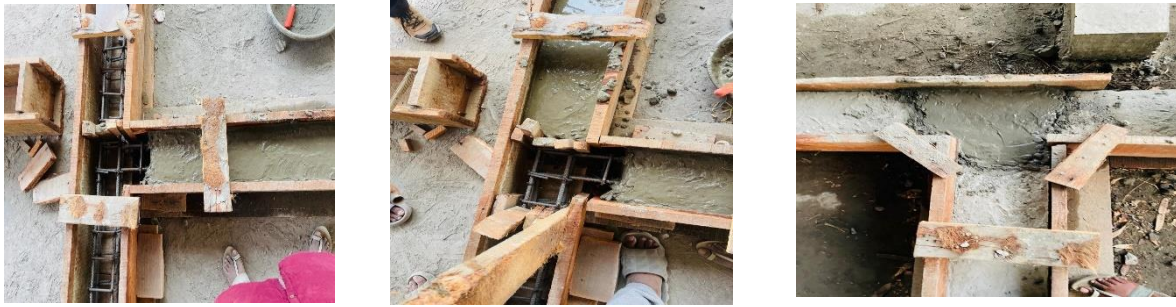
Fig8. Casting of lap joint
