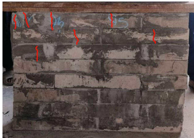
Fig.14 Crack after testing of optimal masonry wall
