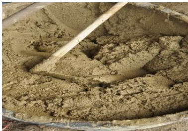
Fig. Soil mixing
