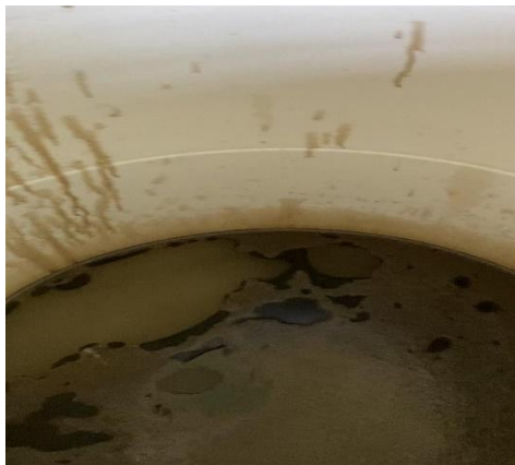
Fig.4.6:Waste Water Stored In Tank
