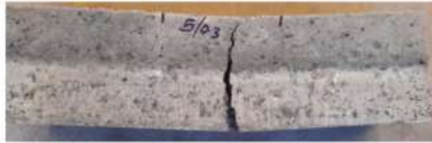
Figure 5 Failure of fiber reinforced concrete
