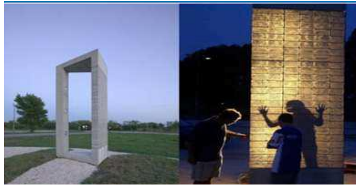
Fig:2 Europe Gate, a 4-meter-high sculpture composed of LitraCon blocks
