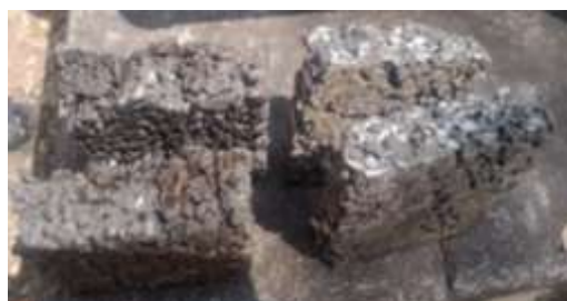
Figure 5 – Flexure failure Blocks Image
