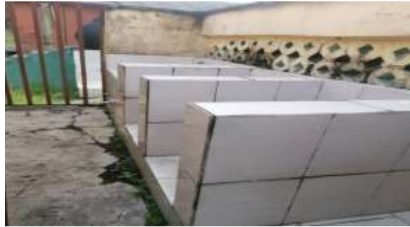
Figure 7 - Toilets and Hand washing Facilities constructed at Egbo Community
