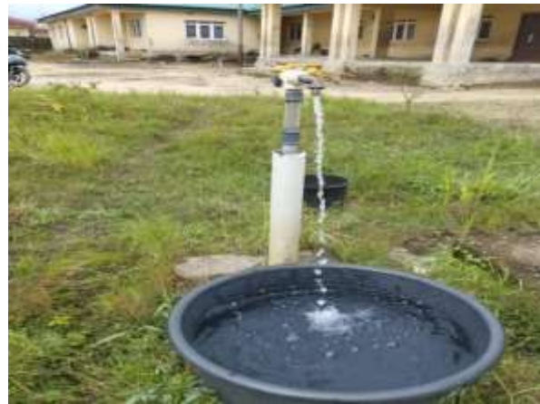
Figure 2 - Functional Borehole at Araya Community
