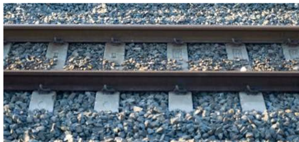
Fig 2 : Traditiona ballast railway track
