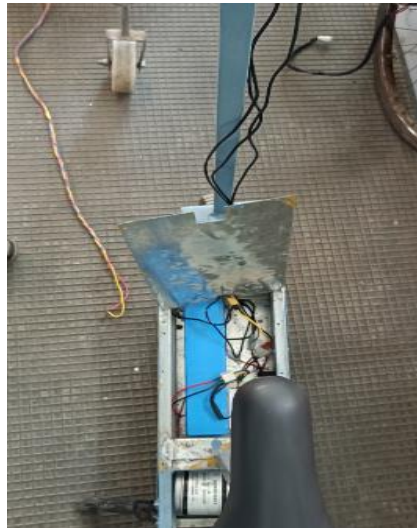
FIGURE 20. Electrical Components Installation and Wiring
