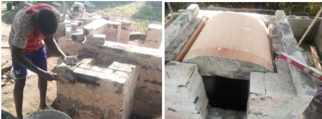
Fig. 6 - Building of the Wall; Chimney and Arc in progress
