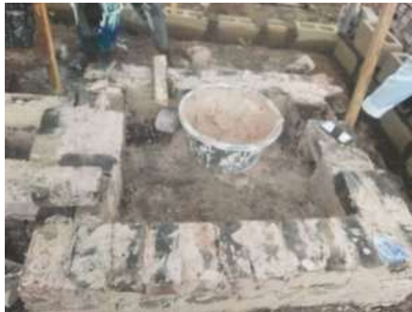
Fig. 4 - Making of the foundation.
