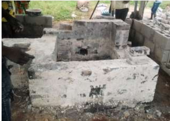
Fig. 5 - The construction of the burner hole on the kiln
