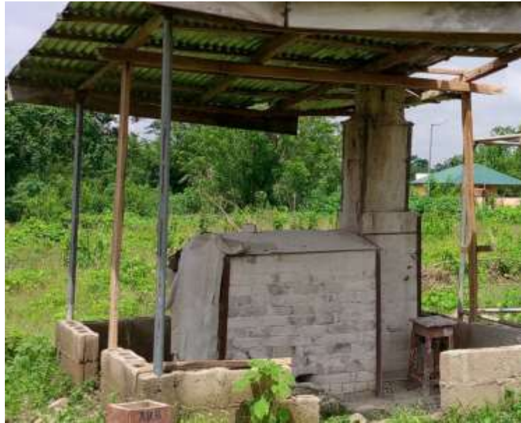
Fig. 7 - Completed Kiln project
