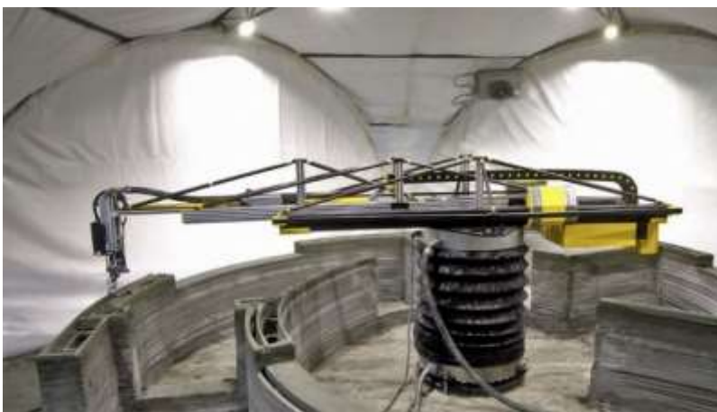
Fig. 1.4: A stationary rotational robotic system for constructing buildings using concrete extrusion. (Dörfler, 2018)
