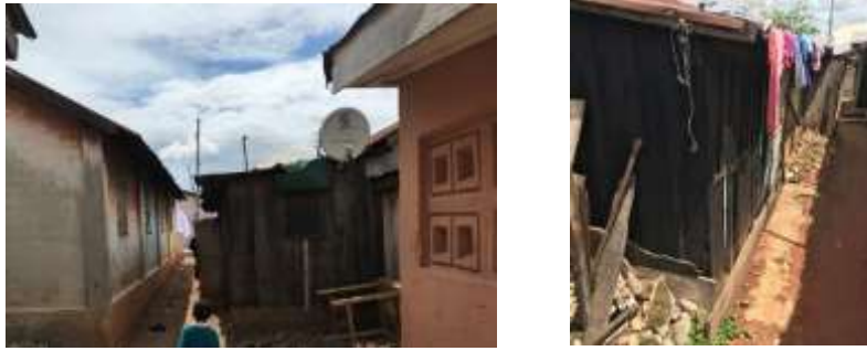
Figure 3.5.1 Extension made to a house blocking access (Source: Author's field study)
