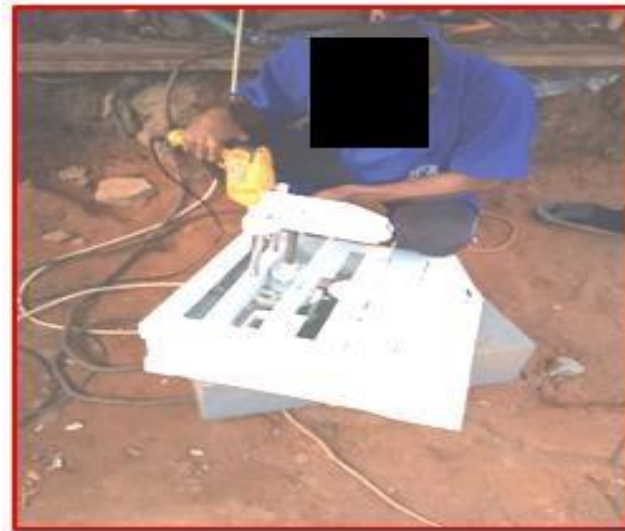
Fig. A1 Construction process in mechanical workshop
