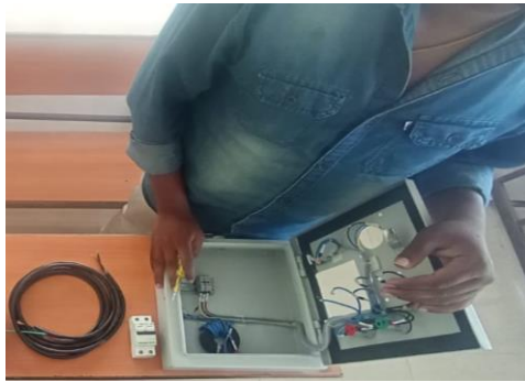
Figure 1 Wiring connections to panel box
