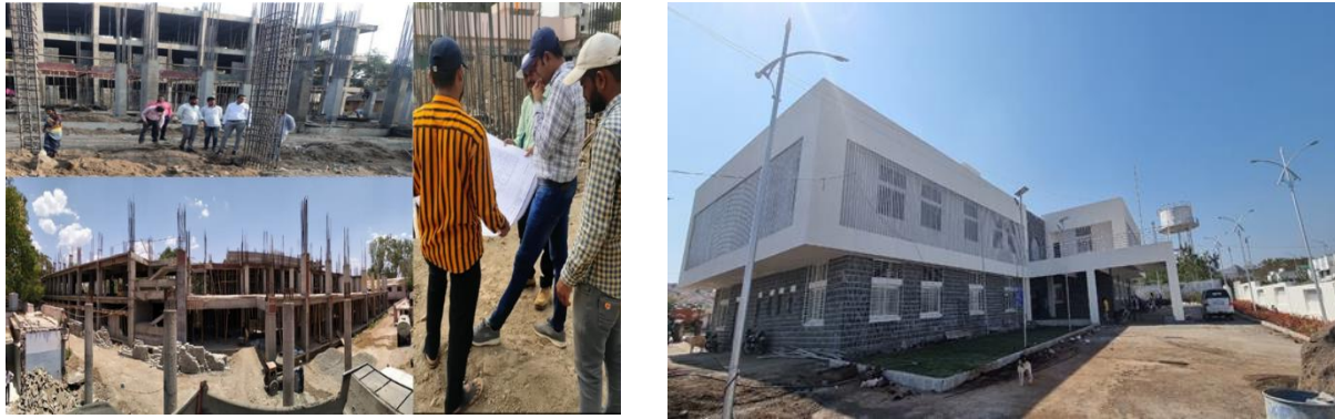
Figure 2: Site Visit Photographs
