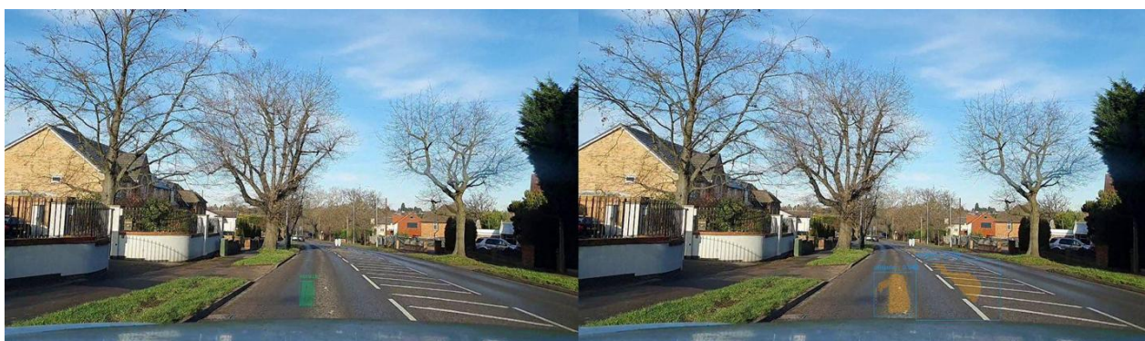
Figure 7. Ground truth on the left and model output on the right for Vertical crack
