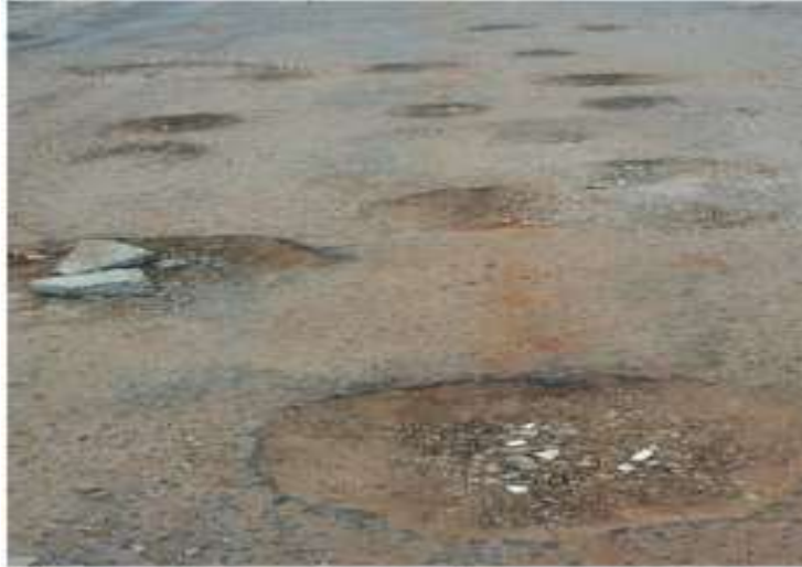
Figure 1. .Pothole Image
