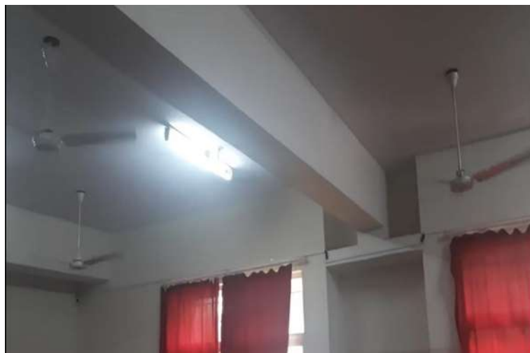
Fig. G - After sensing motion all fans and light of classroom are in ON state (I)
