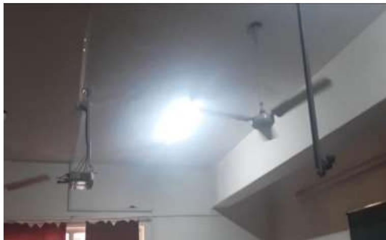
Fig. H - After sensing motion all fans and light of classroom are in ON state (II)
