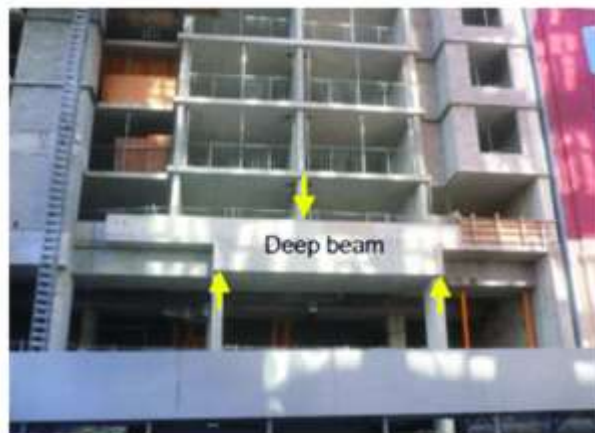
Fig.1 Elements of Deep Beam
