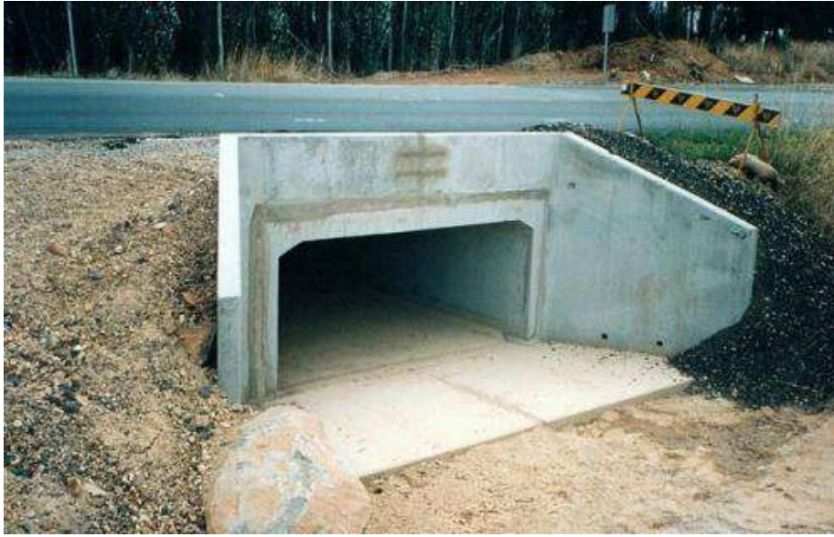
Figure 1 Box Culvert Bridge
