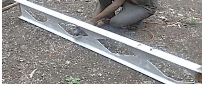
Fig 4 - Grinding of the castellated beam.
