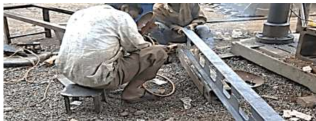
Fig 3 - Welding of castellated beam
