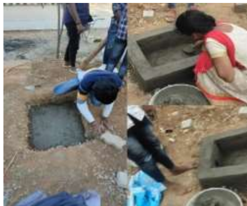
Fig 3.4(b): Construction of Sedimentation Tank
