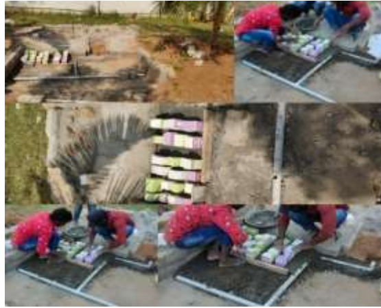
Fig 3.3: Installation of storm drains
